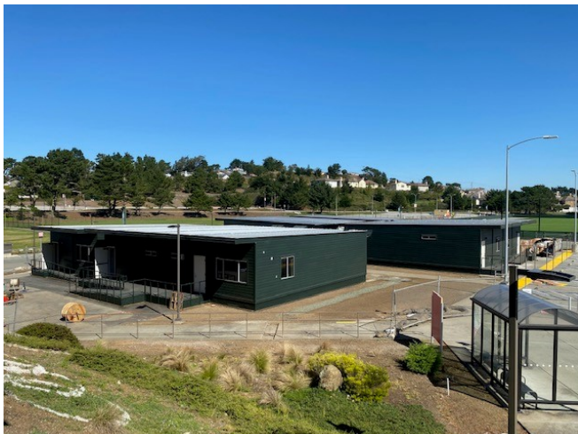
Building B3A-E Portable Replacement Progress
