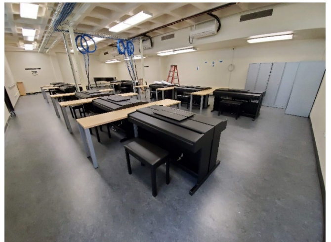
Building 1 Midi/Piano Lab Progress
