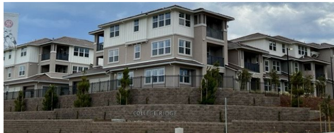
College Ridge Employee Housing Complex at Skyline College
