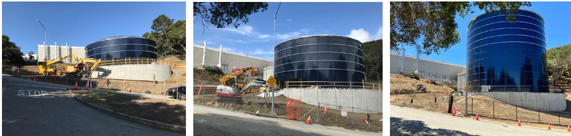
Water Supply Tank Replacement
