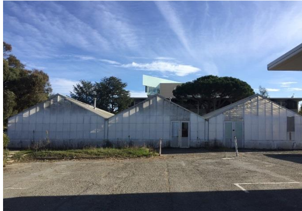
Figure 2. Building 20 greenhouse, viewed facing southeast
