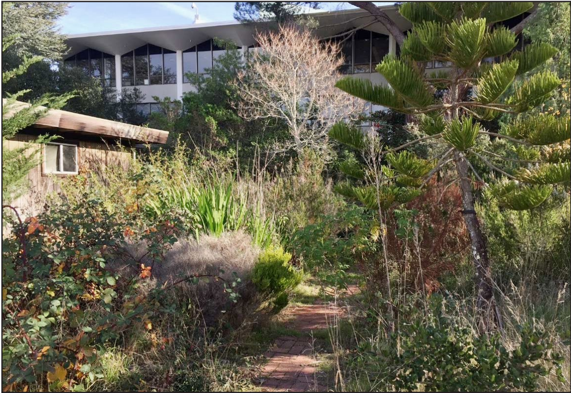
Photo 7. South Garden with Lath House and Building 12 in background (looking east).
