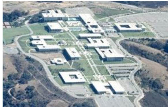
Figure 8. Aerial photograph of CSM campus, c.1965, viewed facing northwest; the Building 20 site is left of center.
