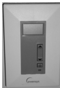
An Override Sensor lets you control the temperature in your area
