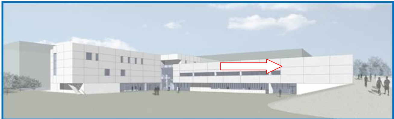
Building 4N as viewed from the Loop Road, looking west.
