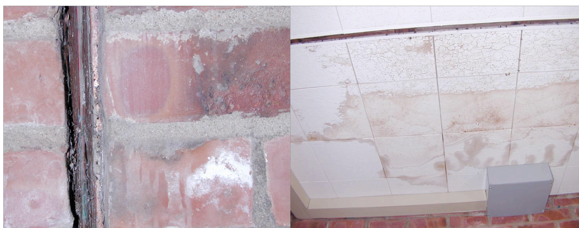
(b) Interior/exterior brick walls
