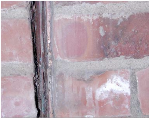
(b) Interior/exterior brick walls
