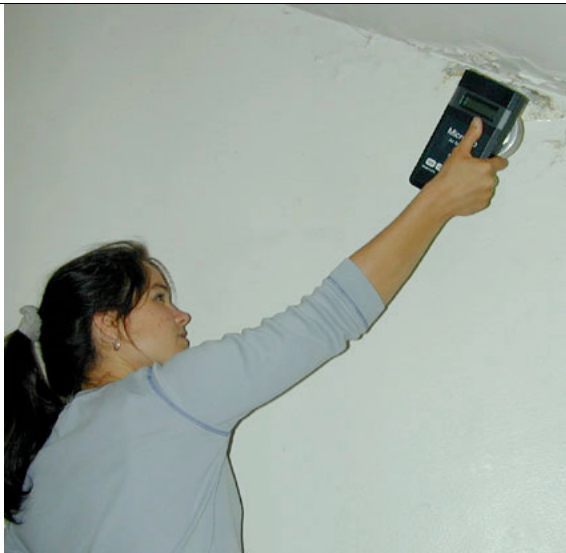
a) Collecting from a water damaged area
